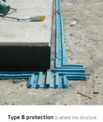
**Type B protection** is where the structure itself acts as a barrier to prevent water ingress. Usually applied during the construction phase of the structure, the protection relies upon the design and materials which are incorporated into the external shell.
