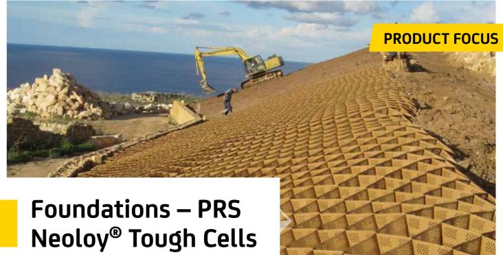
Neoloy® Tough-Cells are a 3D honeycomb geosynthetic made from a nano-polymeric alloy (NPA) for unparalleled performance in terms of stiffness, creep resistance and service life. NPA-based Neoloy® Tough-Cells stabilize soft soil with more engineering, environmental and economic advantages than Soft-Cells (HDPE geocells), chemical additives or any other reinforcement solutions.
