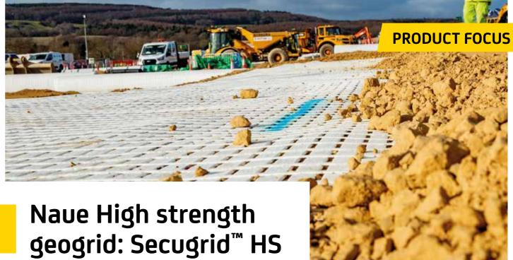
Secugrid™ HS are high strength geogrids. They are laid geogrids made of high tenacity polyester filaments with an extruded polyethylene protective coating and welded junctions.
