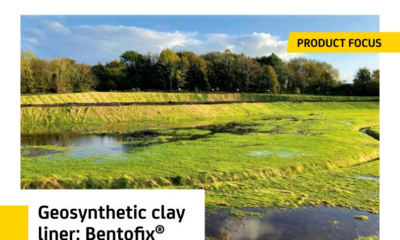
Bentofix®, also known as geosynthetic clay barriers (GBR-C) are needle-punched, reinforced composites that combine two durable geotextile outer layers and a uniform core of high-swelling powder sodium bentonite clay.
