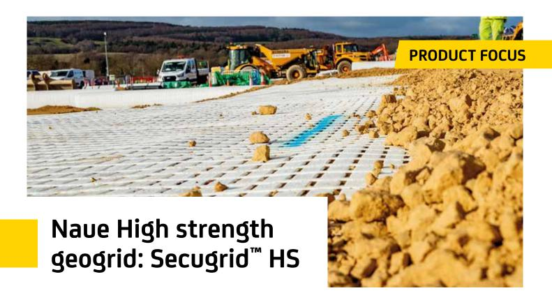
Secugrid™ HS are high strength geogrids. They are laid geogrids made of high tenacity polyester filaments with an extruded polyethylene protective coating and welded junctions.
