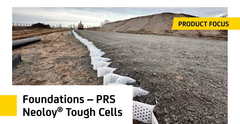
Neoloy® Tough-Cells are a 3D honeycomb geosynthetic made from a nano-polymeric alloy (NPA) for unparalleled performance in terms of stiffness, creep resistance and service life. NPA-based Neoloy® Tough-Cells stabilize soft soil with more engineering, environmental and economic advantages than Soft-Cells (HDPE geocells), chemical additives or any other reinforcement solutions.
